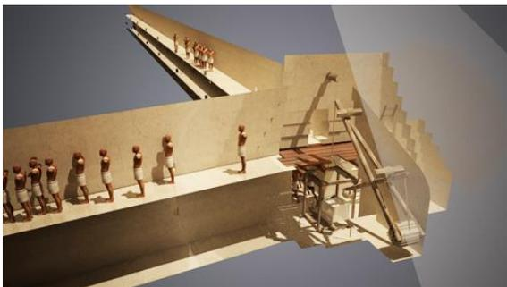
In the corners, the 90° rotations to present the sledges in line with the next section are performed in "rotation rooms" using a lifting machine inspired by the Egyptian Shaduf. In particular, 3D science has enabled us to validate this rotation system, taking into account both mechanical and human aspects. With this system, it takes around two minutes to rotate a block.
