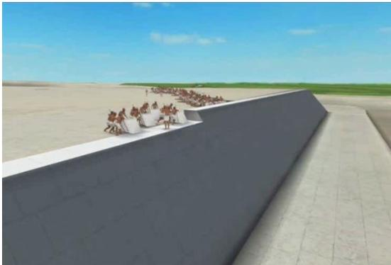
By building from the inside-out, the faces are completed as construction progresses, so there's no need to come back at the end of the project to resurface 84,000m<sup>2</sup> of faces, which means years of extra work.
