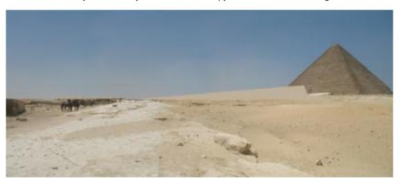
The original ramp linking the port to the base of the exterior ramp of the construction site for the pyramid of Khufu; forming an angle of 80°, this latter ramp (shown in beige at the centre of the photograph) continues on from the first ramp with a comparable slope. The total length of the two ramps is about 970 m and they rise 83 m between the level of the port and the level of the base of the King's Chamber, an average slope of 8.55%.
