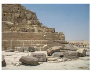
On the left, the central part of the eastern base of the pyramid; to the right, the north-east corner. The first four courses are "sculpted" directly into the bedrock or from blocks cut slightly set back from the face and then moved forward to the edge.
