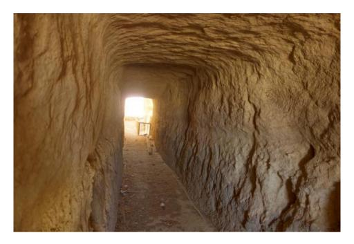
The tunnel crosses the Chaussée Monumentale a few meters below it. Traces of stagnant water are clearly visible on the side walls and at the bottom.
