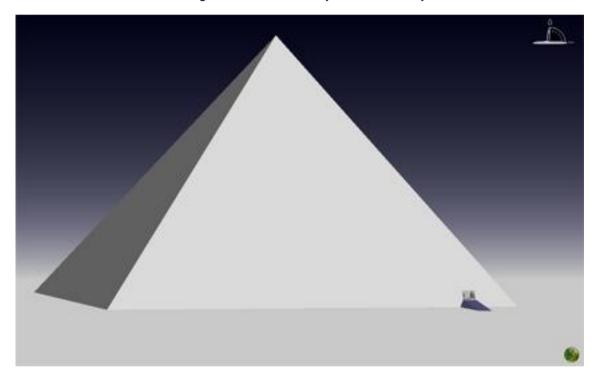
The pyramid of Khufu was constructed from the inside as far as the top, the facing blocks made of Tura limestone having already been fashioned in their final form prior to being laid. No openings to the outside were retained during construction, except for the entrance to the interior ramp on the south face, near the south-east corner.
