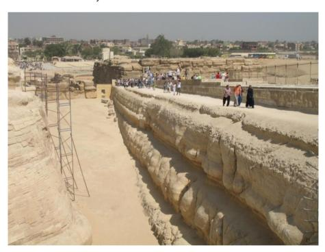
The space between the pit and the masonry of the monumental roadway is heavily eroded at the top; there is also a marked sense of run-off erosion at the bottom of the pit.
