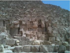
The positions of the blocks are very curious; some parts have been sealed by rubble and cement mortar, while on each side of this area the stone-work is matched and regular. We also found recent stone-work that came to the fore in places.
